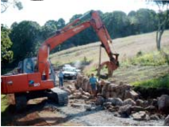
Paul Morgan Constructions worked with Tom Condon's team to construct rock walls from loose rock found onsite.
