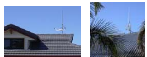
Rooftop aerials (above) connect subscribers to broadband via a wireless network.
