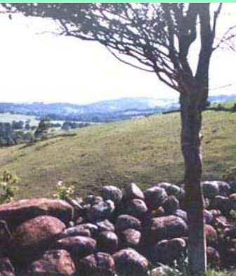
Original stone walls (bottom) the design model for new retaining walls throughout the community
