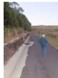
(Left) The Kahlert's landscaped waste water treatment system.
